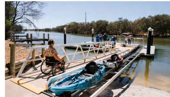
g All abilities paddle launch facility
